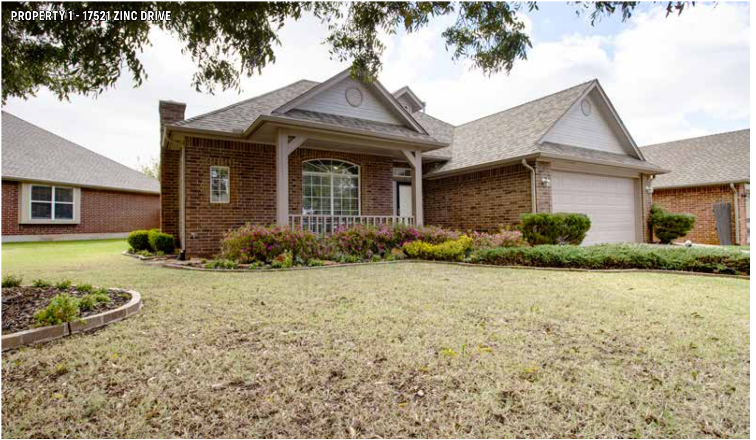
PROPERTY 1 - 17521 ZINC DRIVE
