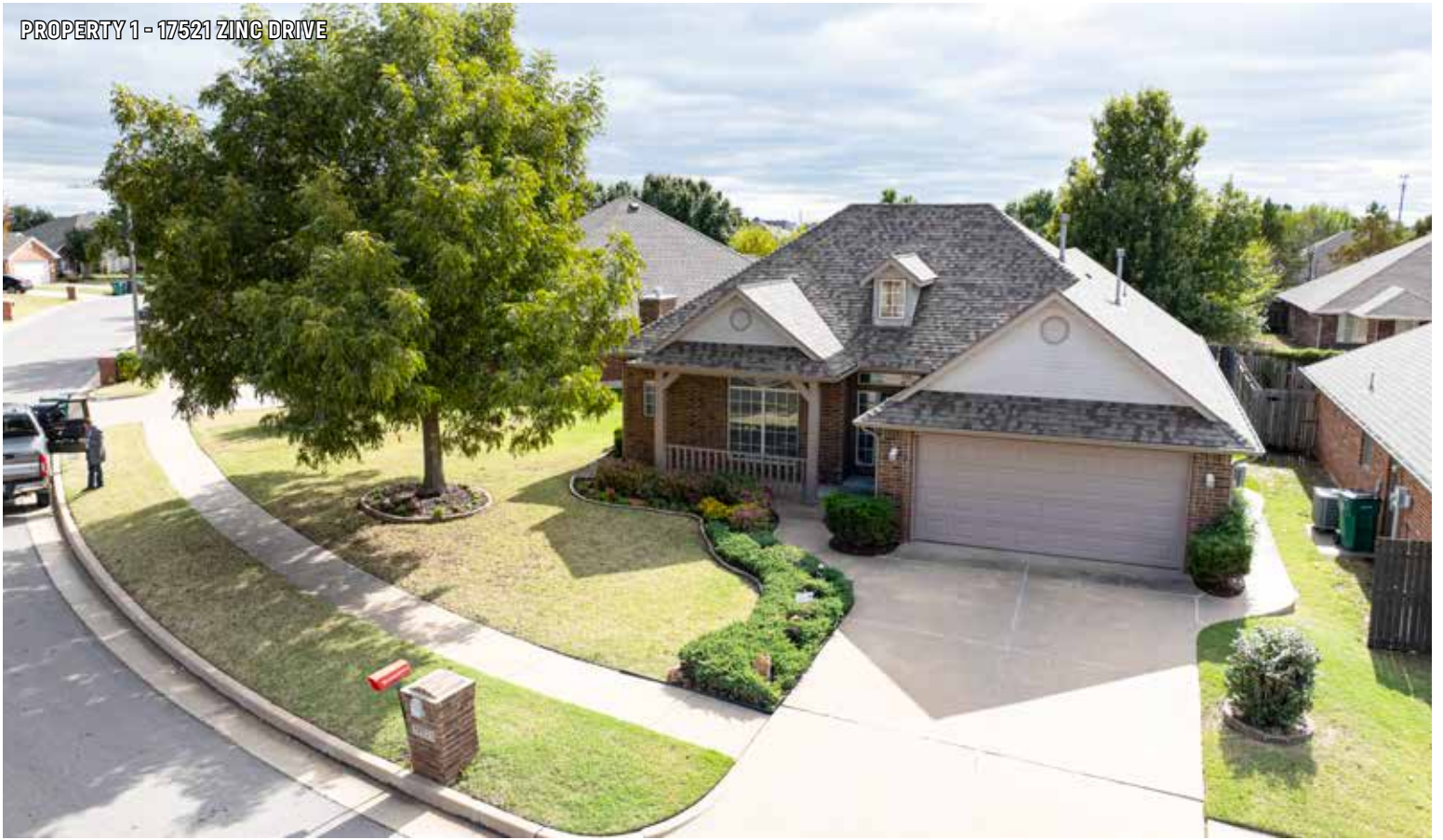
PROPERTY 1 - 17521 ZINC DRIVE
