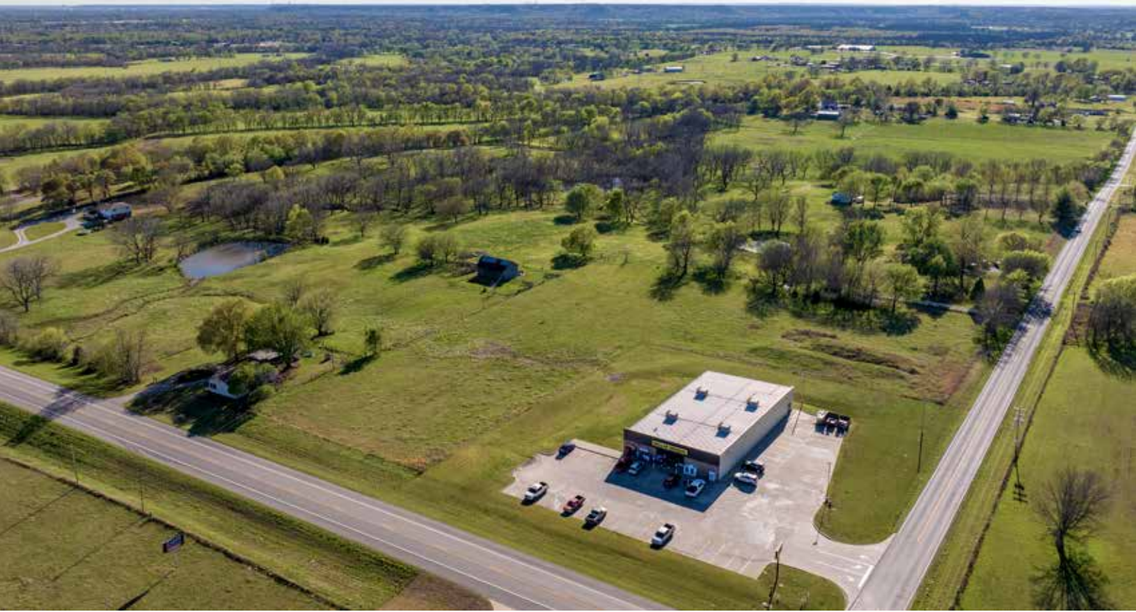
Northwest Corner View
