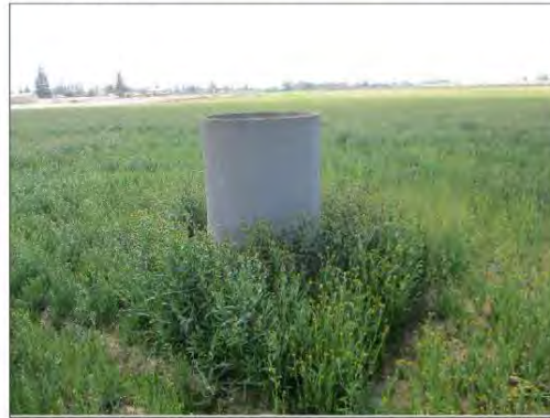
6. Concrete standpipe on the subject property
