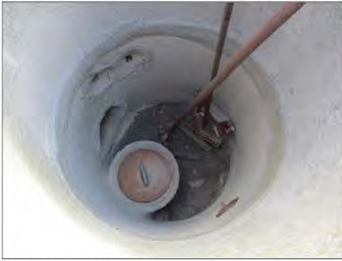
7. Concrete standpipe
