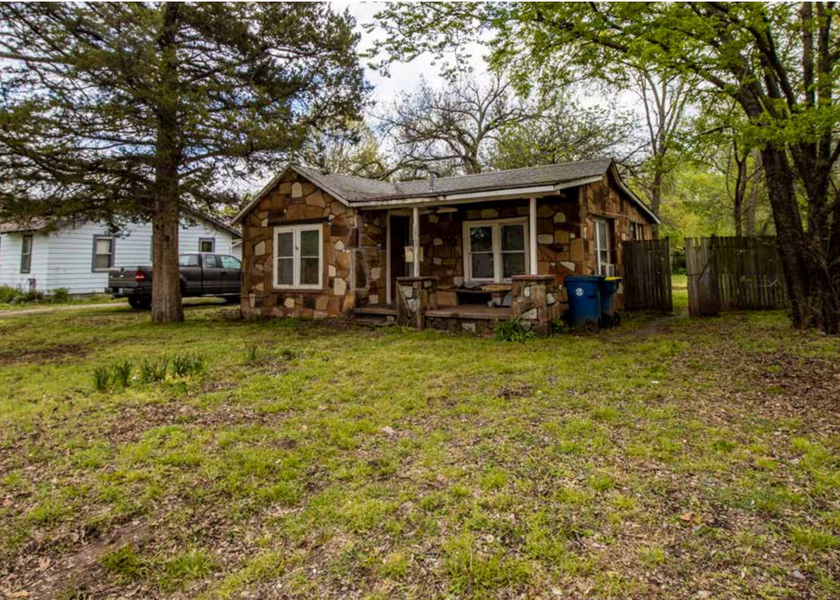
TRACT 10: 1503 S. Springfield St – 1Bd, 1Ba rock exterior home, new roof in 2009, HUGE back yard fully fenced, 597 Sq. Ft.
