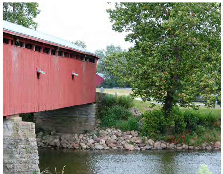
Figure 3.1: The Great Miami River flowing under the Eldean Covered Bridge
