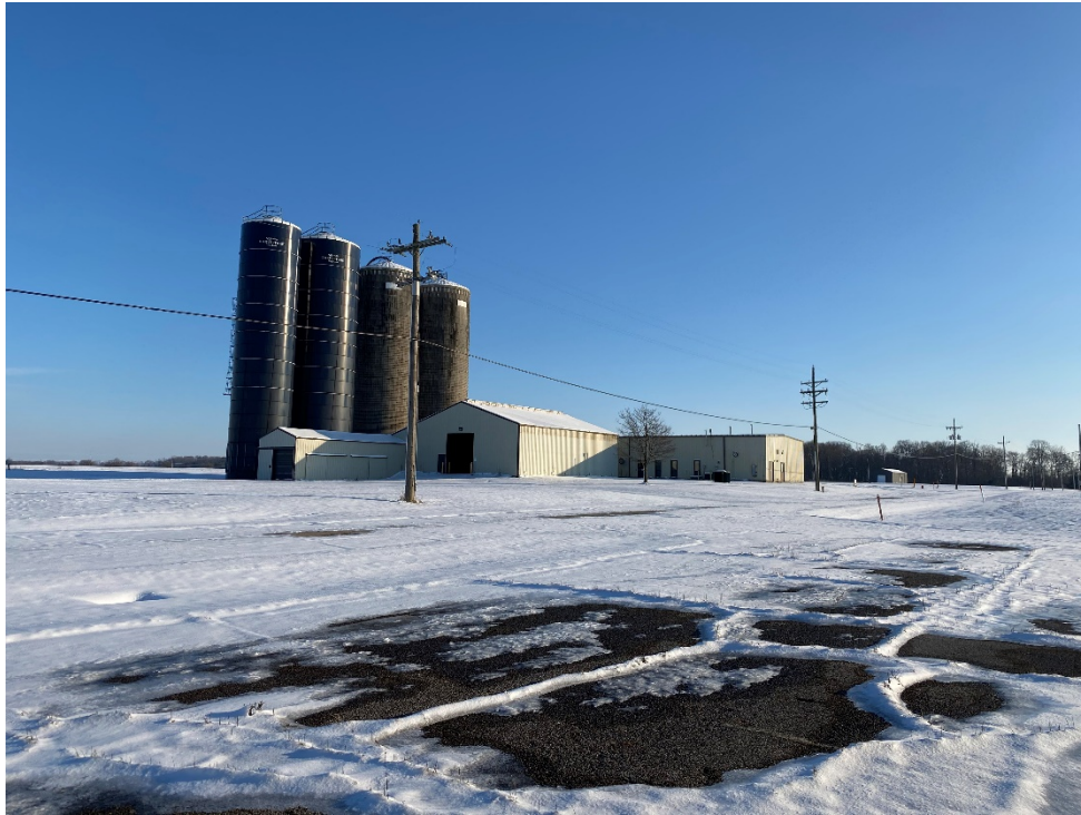
Photo 17 - View of Building 234 and grain silos
