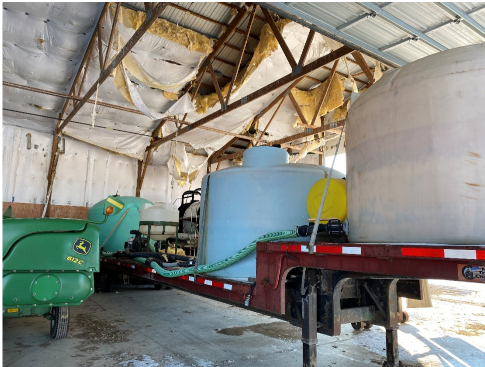
Photo 3 - View of tank storage on the West Farm
