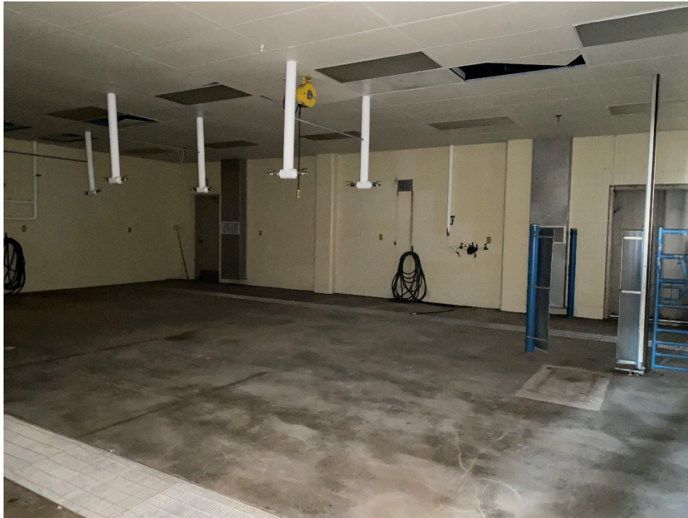
Photo 15 - View of old lab area in Building 293
