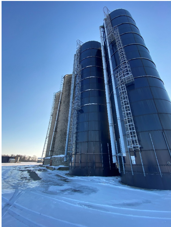
Photo 20 - View of grain silos
