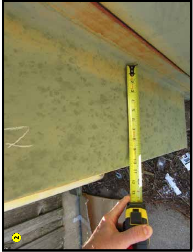
- View of Hail Spatter on Electrical Transformer
